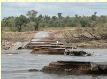
Roads washed out to Halls Creek
