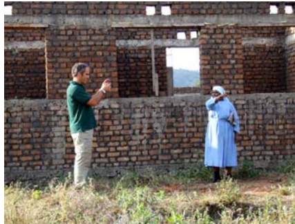
Gavan with Sister Zabibu by the partially built hostel
